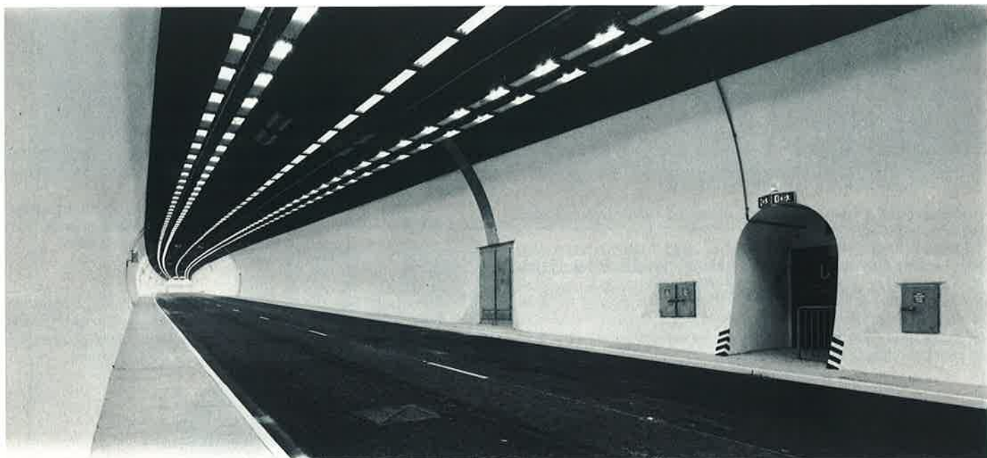
Round Hill Tunnel, UK
