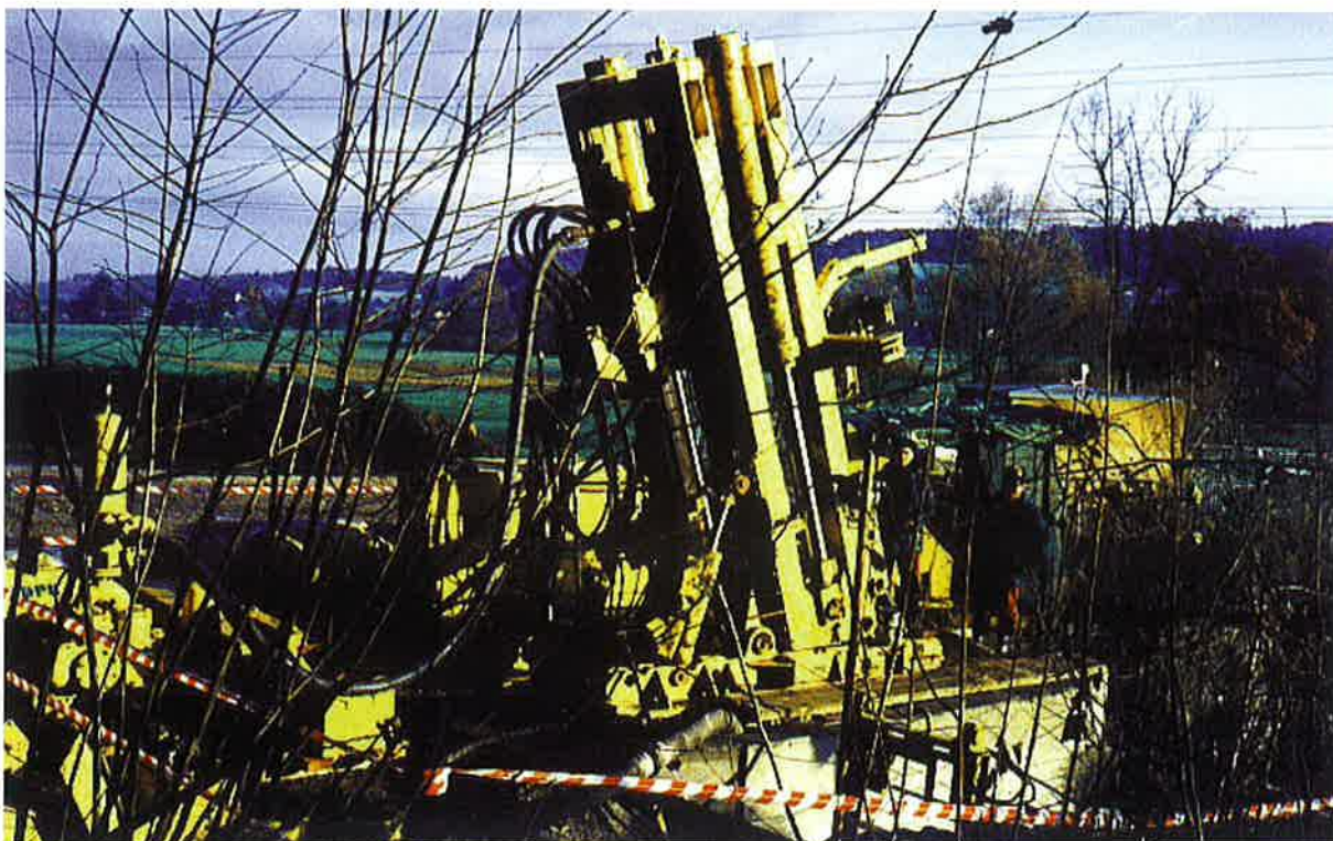
Obr. 8 Pohled na staveniště Fig. 8 View of Working Site
