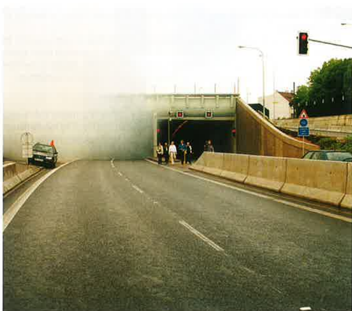
Obr. 5 Portál tunelu Husovice asi 7 minut po vzniku simulovaného požáru The Husovice tunnel portal 7 minutes after the simulated fire had started
