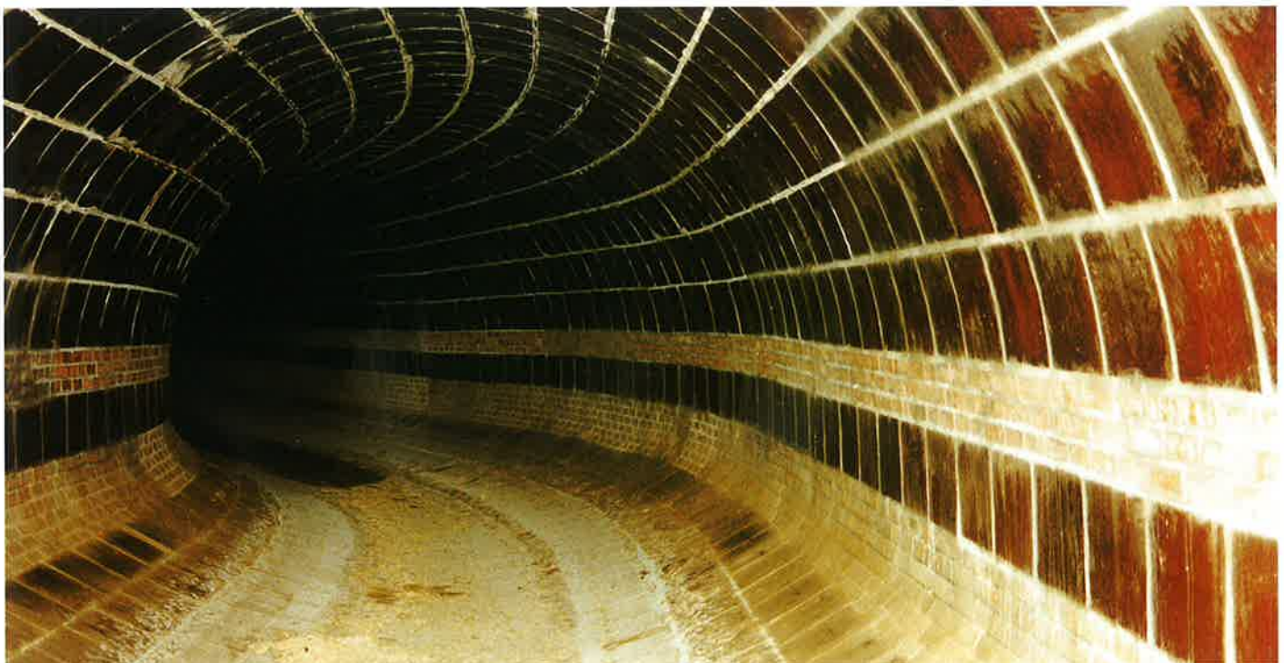
Obr. 7 Tlakový profil kmenové stoky v prostoru pražské zoo Mouth-shape profile of the main sewer in the area of the Prague zoological garden
