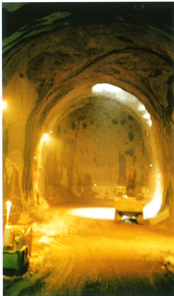
Obr. 3 Kaverna vetracej stanice Flossgraben The Flossgraben ventilation station cavern
