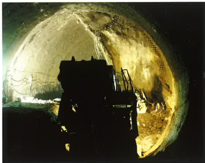
Obr. 5 Ražba pilíře Fig. 5 The driving and concrete casting of the pillar
