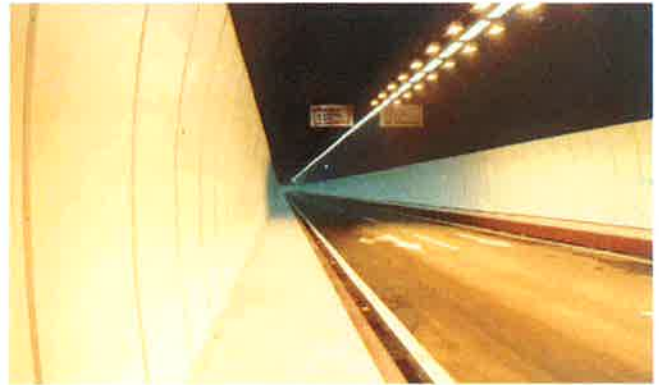
Tunnel "CHONGQING", China
