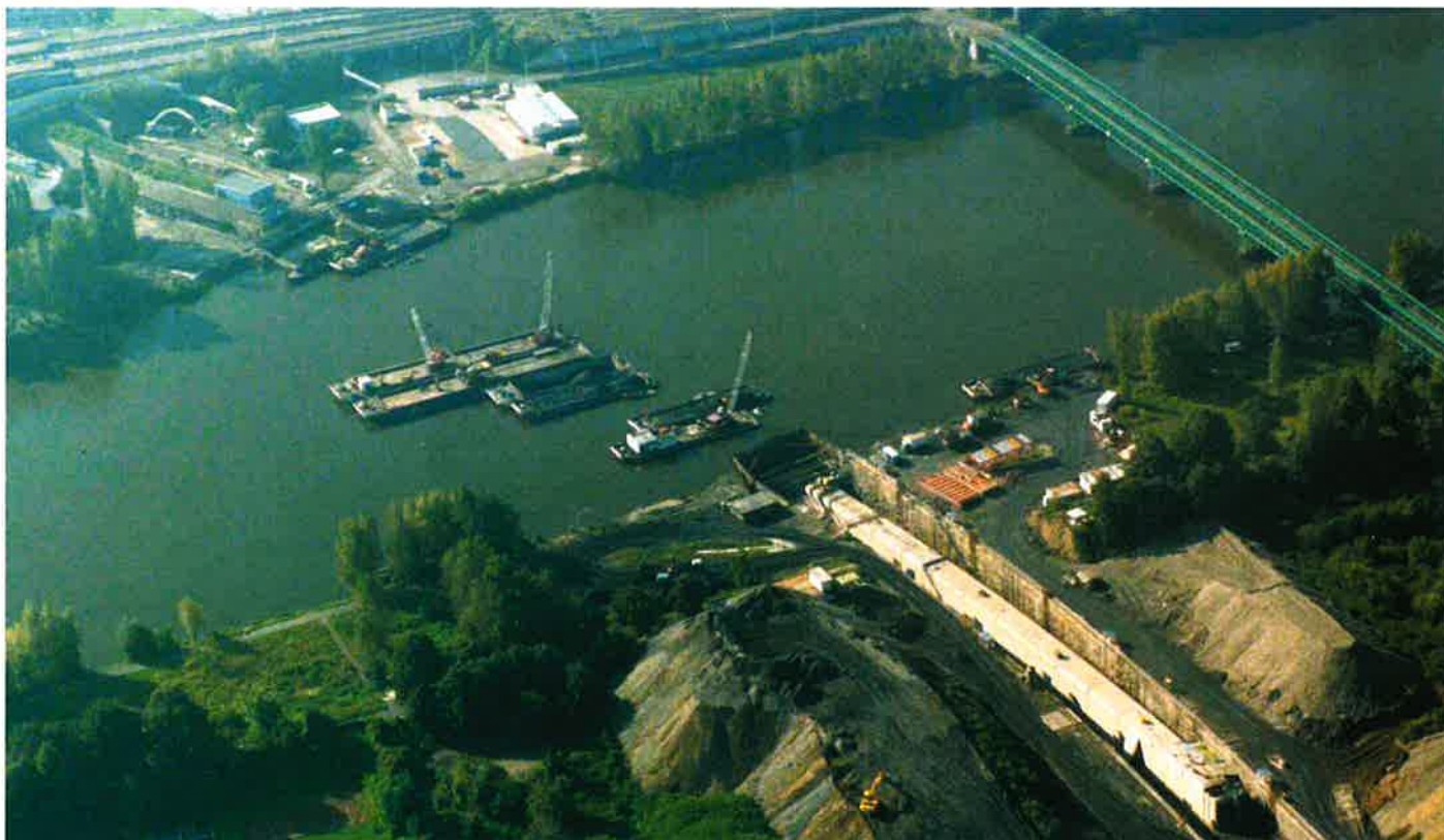
Obr. 3 Hotový tunel v doku Fig. 3 Completed tunnel in the dry dock
