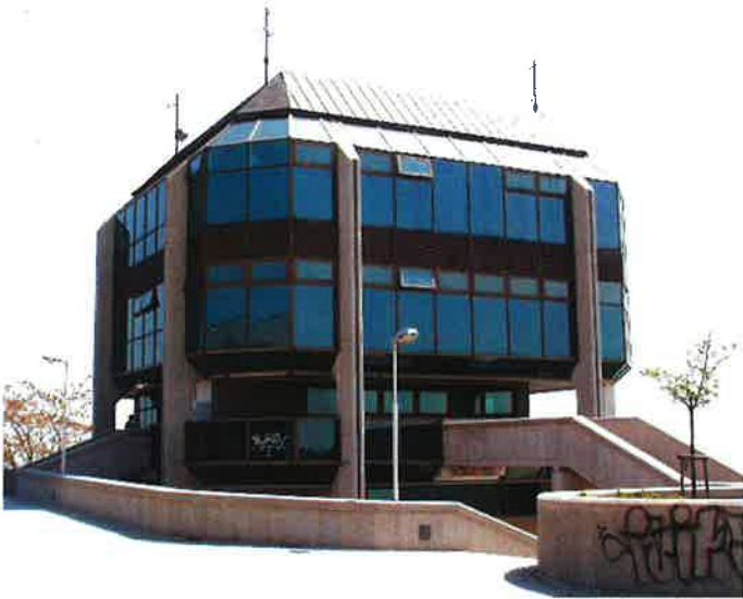
Obr. 2 Budova velínu SAT Fig. 2 SAT control building
