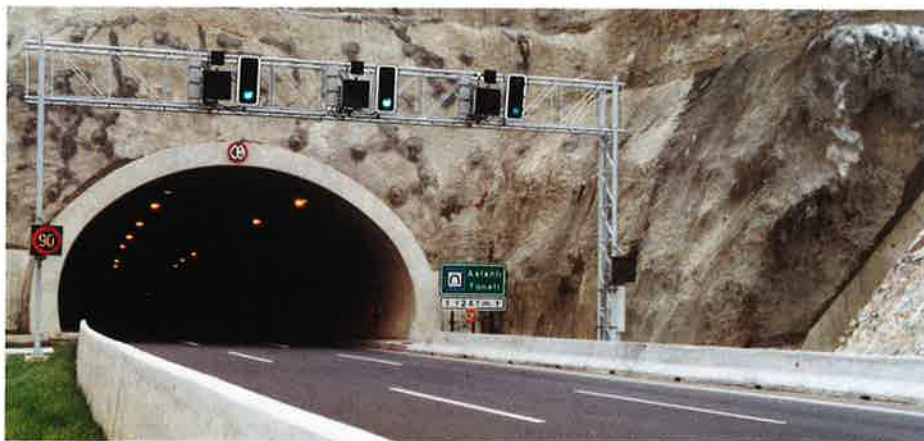
Obr. 1 Vjezd do tunelu Aslanli ve směru na Gaziantep po uvedení systému do provozu Fig. 1 Access into the Aslanli tunnel in the direction towards Gaziantep after putting the system into operation
