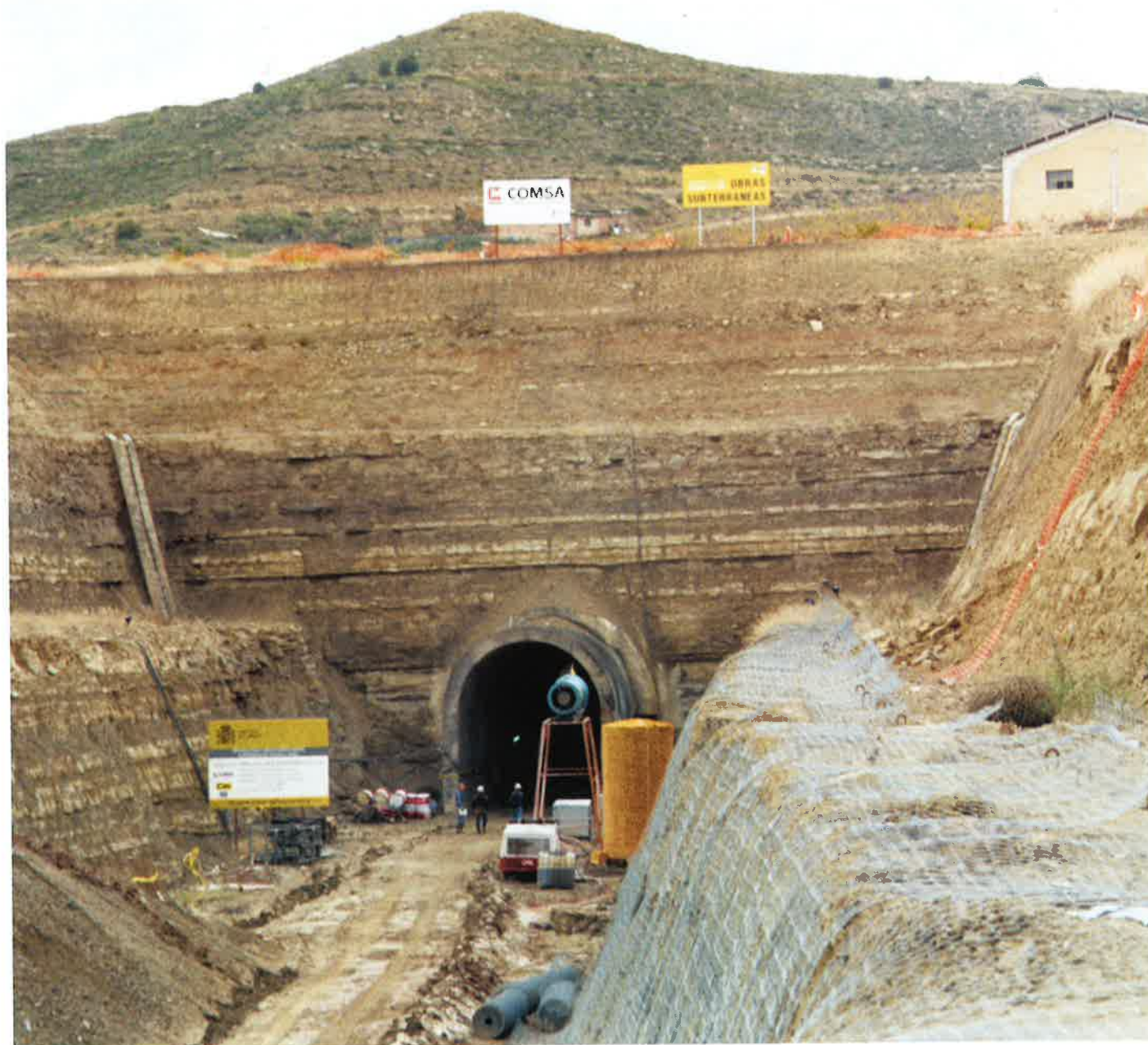
Obr. 4 Detail portálu tunelu Fig. 4 Detail of the tunnel portal
