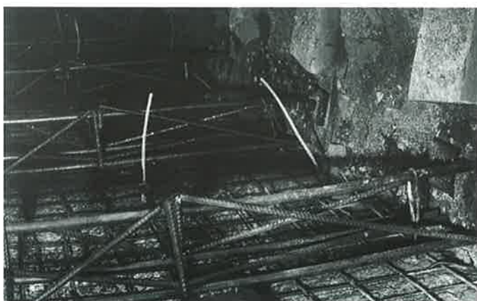
Obr. 4 Sychrovský tunel Fig. 4 The Sychrov tunnel
