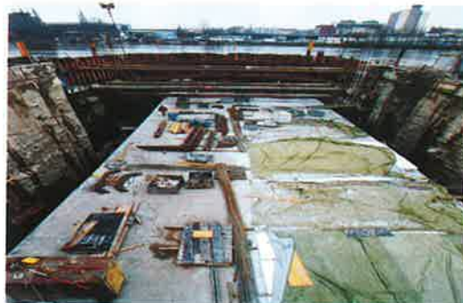
Realizace trasy metra IVC 1 Construction of Prague underground, line IVC 1
