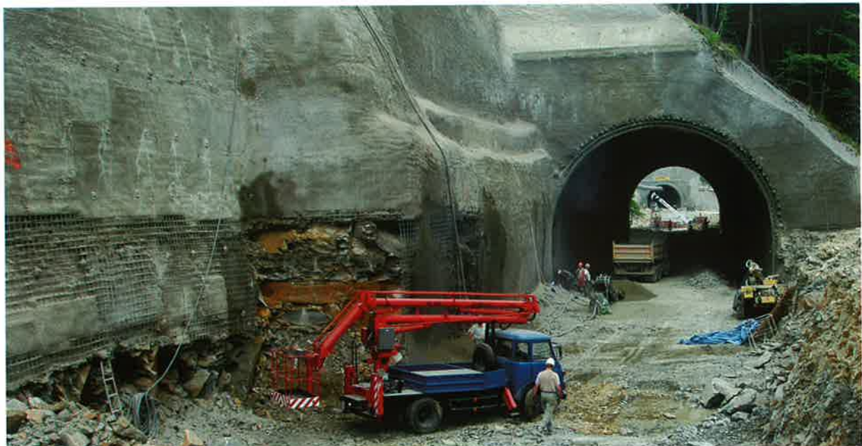
Obr. 6 Dokončená ražba tunelu Krasíkov II Fig. 6 Krasíkov I tunnel excavation completed
