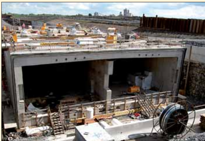
Obr. 1 Stavba tunelu Limerick Fig. 1 Limerick tunnel construction
