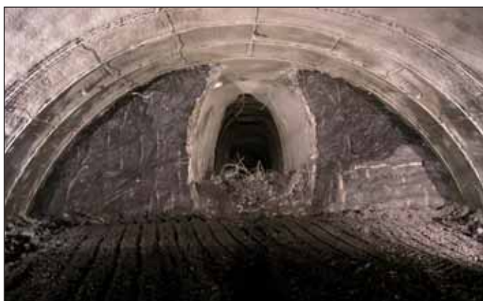
Obr. 3 Průzkumná štola v profilu tunelu 3PT Fig. 3 The exploration gallery within the profile of the 3LT
