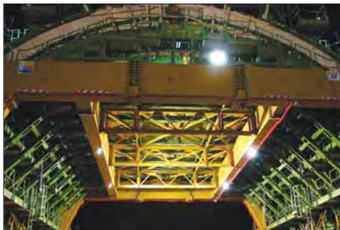
Obr. 4 Samohybne oceľové debnenie hornej klenby Fig. 4 Self-propelled formwork for the upper vault
