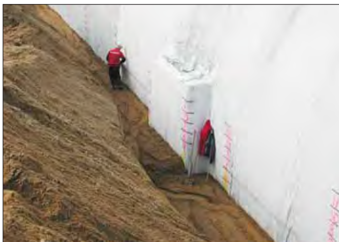
Obr. 2 Postupné obsypávání tunelu podle rysek na geotextilii Fig. 2 Gradual backfilling of the tunnel according to marks on the geotextile
