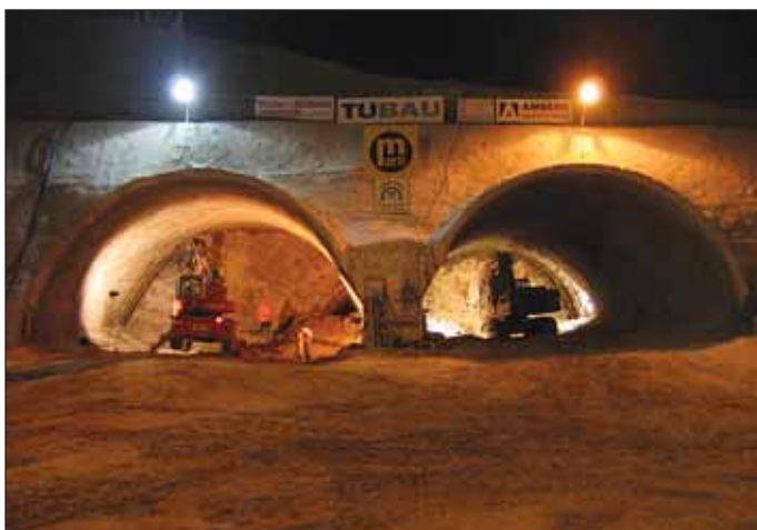
Obr. 4 Razenie prebiehalo súčasne v oboch tunelových rúrach Fig. 4 Driving operations were carried out simultaneously in both tunnel tubes
