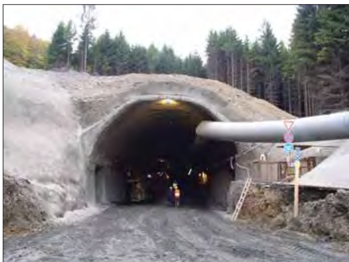
Obr. 14 Ražba tunelu Malá Huba pod provizorní klenbou Fig. 14 Driving the Malá Huba tunnel under the temporary vault
