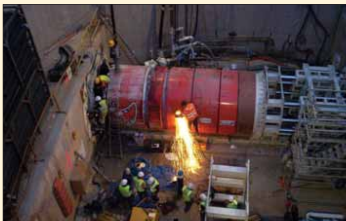
Obr. 1 Pohled do šachty s mikrotunelovacím strojem ISEKI Unclemole CTP Fig. 1 View down the shaft with ISEKI Unclemole CTP microtunnelling machine
