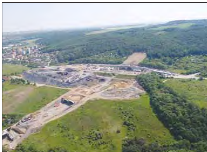
Obr. 3 Tunely SOKP 513 Fig. 3 Tunnels on PCRR 513 construction lot
