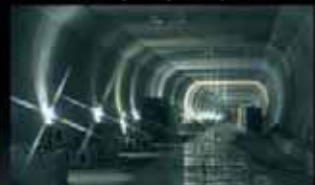
Královo Pole tunnel, Brno ring road
