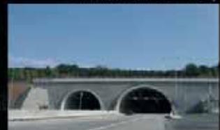
Cholupice tunnel, Prague ring road
