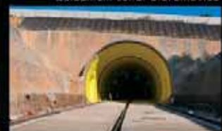
Olbramovice railway tunnel
