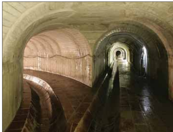
Obr. 6 Rozplet štol 1 a štol 2 Fig. 6 Bifurcation of gallery 1 and gallery 2
