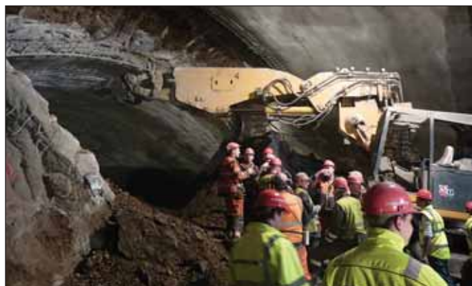
Obr. 4 Prorážka severního tunelu Brusnice 11. 4. 2011 Fig. 4 The breakthrough of the northern tube of the Brusnice tunnel
