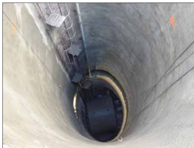
Obr. 8 Šachta Š1 po opláchnutí tlakovou vodou a vzduchem Fig. 8 Shaft Š1 after washing with high-pressure water and air
