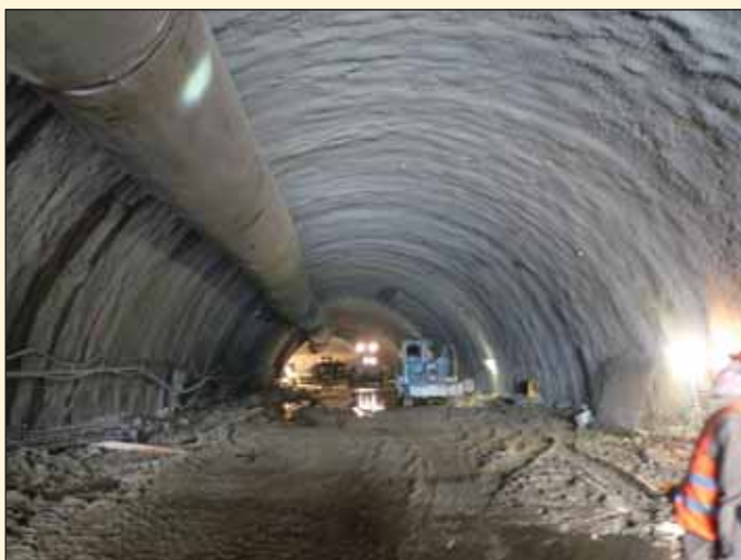
Obr. 5 Ražba tunelu Tomice II Fig. 5 Tomice II tunnel excavation
