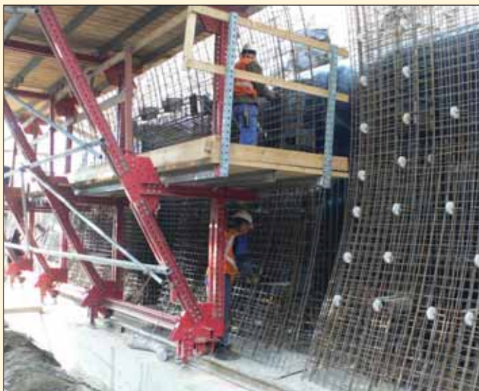
Obr. 3 Montáž samonosné výztuže tunelu Votice Fig. 3 Assembly of the self-supporting reinforcement of the Votice tunnel
