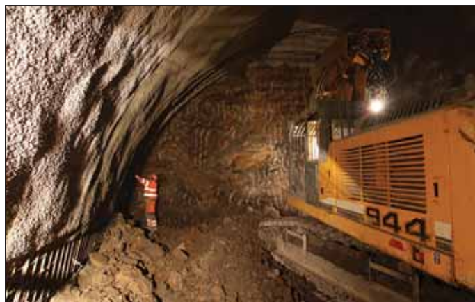
Obr. 3 Čelba jižního tunelu Brusnice Fig. 3 Excavation face in the southern tube of the Brusnice tunnel
