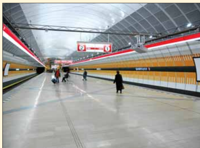
Obr. 2 Jednolodní stanice Kobylisy na trase C (2004) Fig. 2 Kobylisy single-span station on the Line C (2004)
