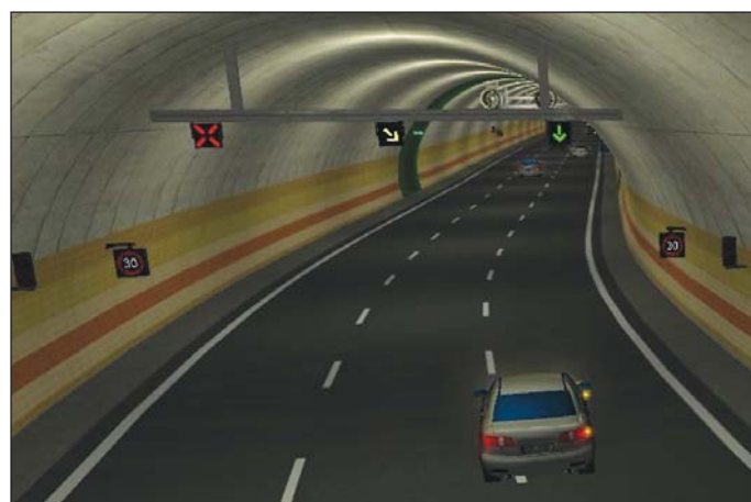
Obr. 5 Místo v tunelu s PDZ (S1, S8 a B20a) Fig. 5 Place in a tunnel with variable traffic signs (S1, S8 and B20a)
