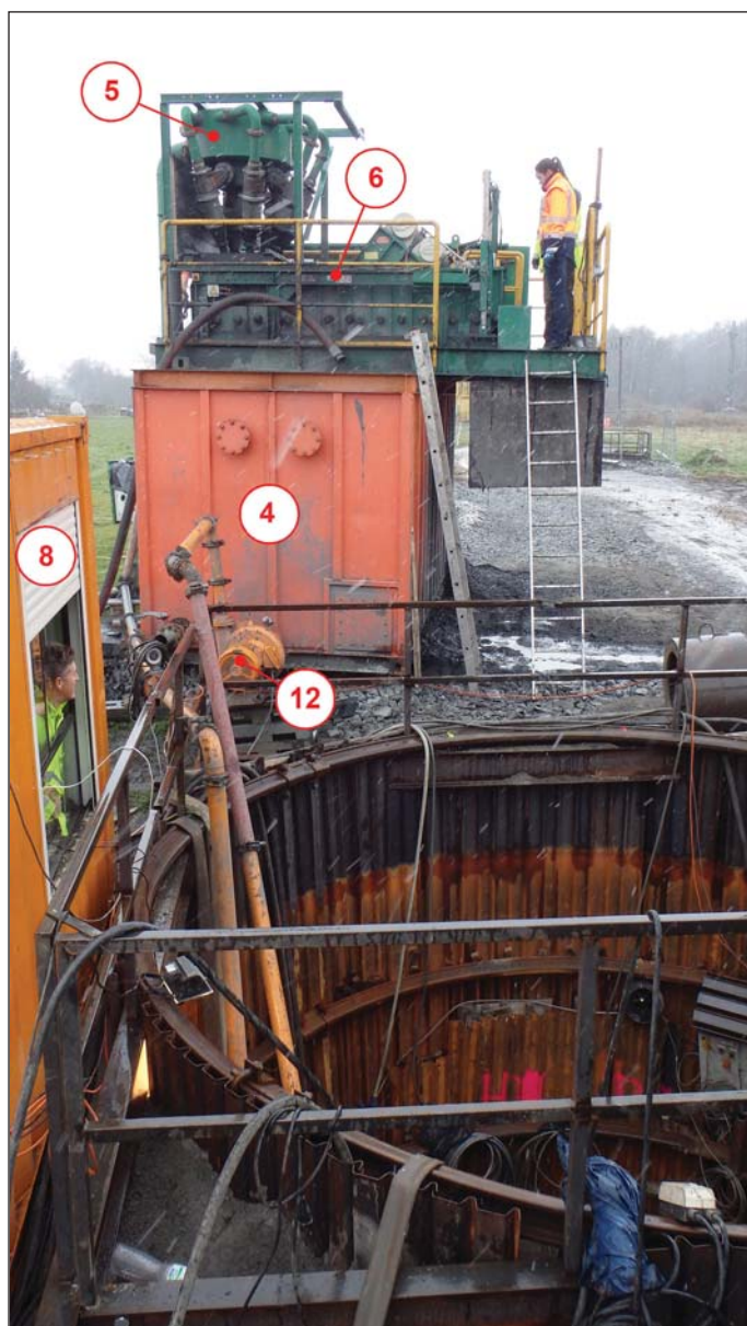
Obr. 6 Povrch – velín ⑧, separace, šachta Fig. 6 Surface – operation cabin ⑧, separation plant, shaft
