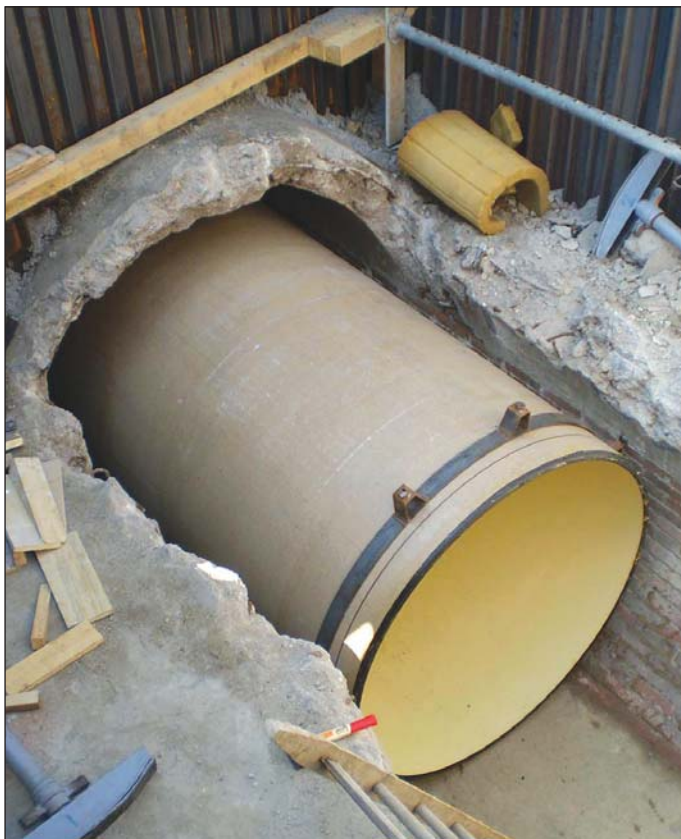
Obr. 9 Trubka GRP ve štolě – Troja Fig. 9 GRP tube in the gallery – Troja
