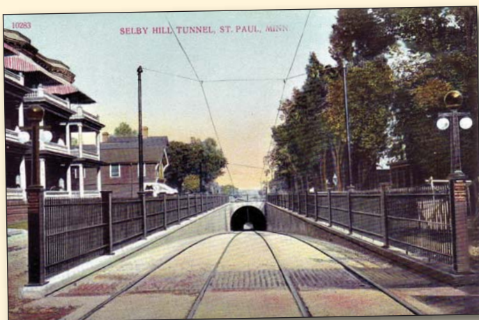
Obr. 6 10283 Selby Hill tunnel, St. Paul, Minnesota
