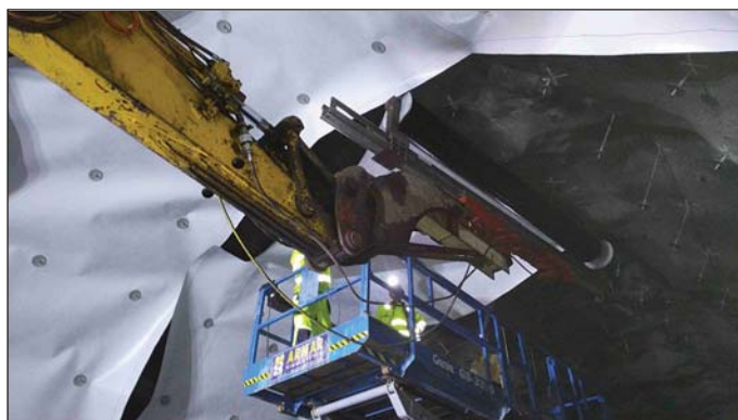
Obr. 8 Instalace polyetylenové membrány Fig. 8 Installation of the polyethylene membrane
