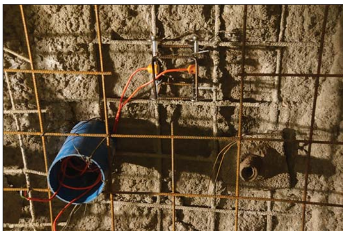
Obr. 10 Osazené tenzometry – tunel Sudoměřice Fig. 10 Tensometers installed in the Sudoměřice tunnel
