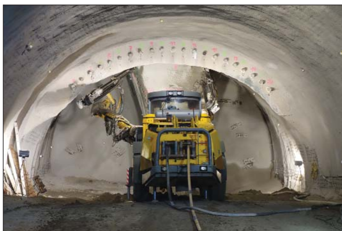
Obr. 7 Ražba tunelu Sdružení Tunel Spitzenberg + trasa BA2 Spitzenberg Tunnel + BA2 Route Consortium Fig. 7 Tunnel excavation
