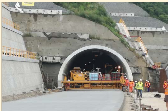
Obr. 2 Tunel Žilina – cementobetónová vozovka Fig. 2 Žilina tunnel – concrete roadway
