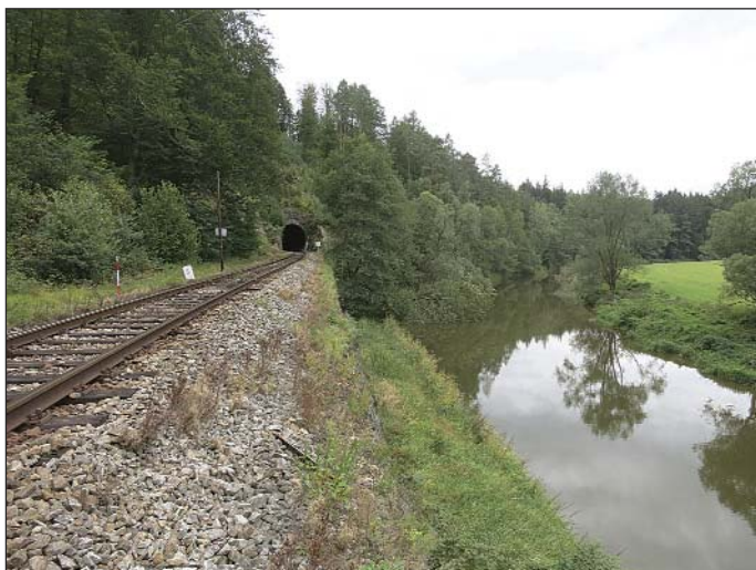
Obr. 1 Pohled na vjezdový portál tunelu Podhradský Fig. 1 A view of the entrance portal of the Podhradský tunnel
