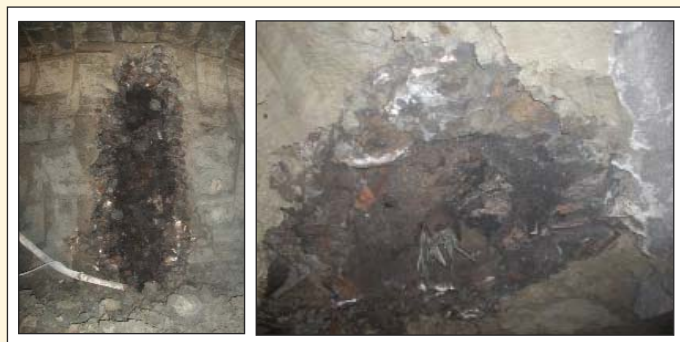
Obr. 6, 7 Studna nafáraná v kalotě jižního tunelu Fig. 6, 7 A well stricken at the southern tunnel tube top heading
