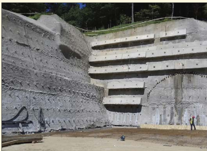
Obr. 3 Tunel Prešov Fig. 3 Prešov tunnel
