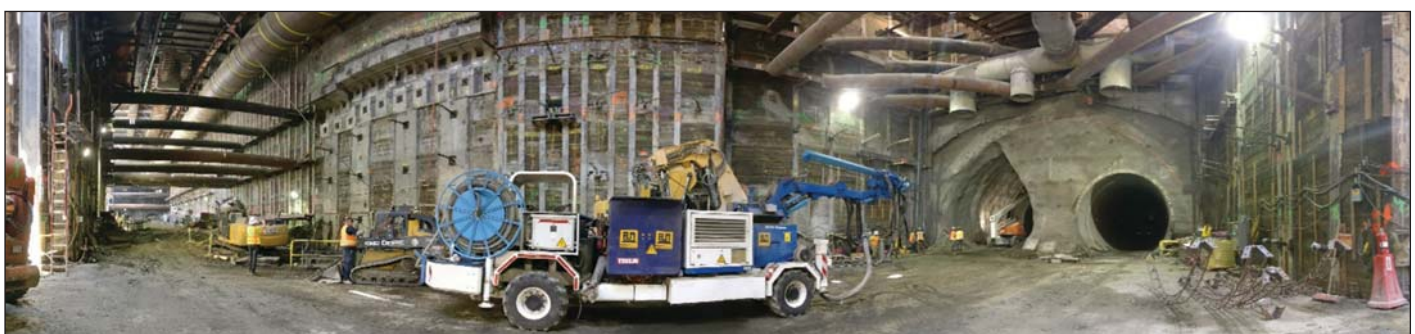
Obr. 3 Ražba kaverny, panoramatický pohled z hloubené stanice Historic Broadway Fig. 3 SEM cavern construction, panoramic view from Historic Broadway Station cut-and-cover
