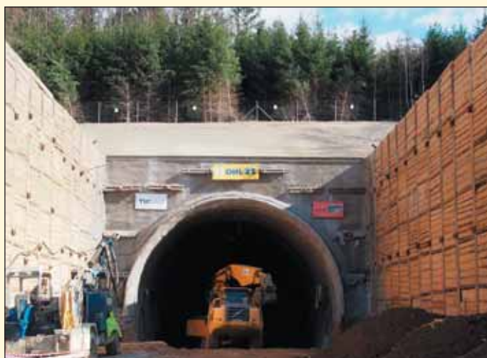
Obr. 1 Tunel Deboreč Fig. 1 Deboreč tunnel
