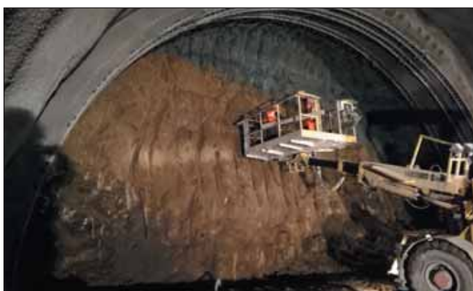
Fig. 5 Pohled na geologii čelby ve třídě VT Vc Fig. 5 A view of geology at excavation face, excavation support class VT Vc
