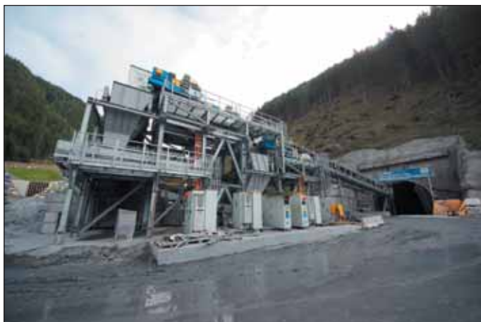
Obr. 5 Deponie Padastertal pro 7,7 mil. m 3 rubaniny Fig. 5 Padastertal stock pile for 7.7 million m 3 of muck
