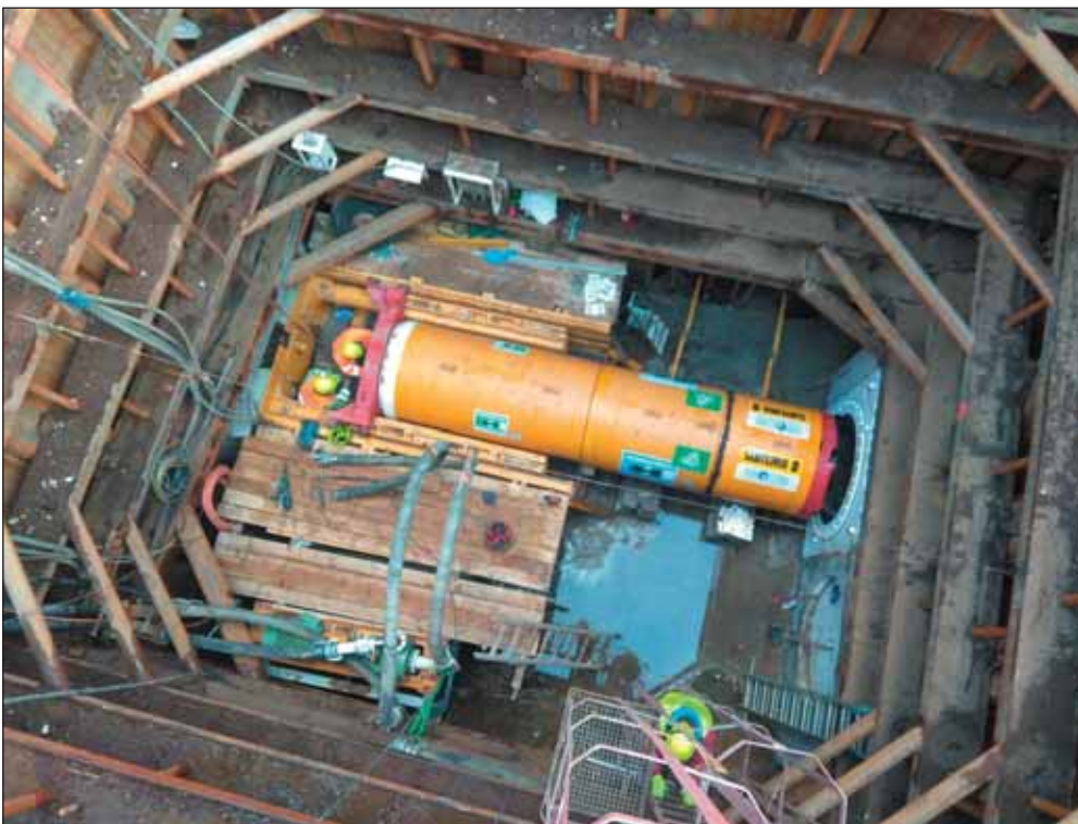
Obr. 7 Razičí štít AVN800XC-A a back-up roura Fig. 7 AVN800XC-A tunnelling shield and back-up pipe
