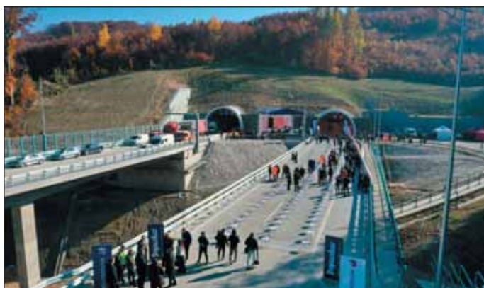
Obr. 1 Priestor pre hostí slávnosti na západnom portáli tunela Prešov Fig. 1 Space for guests at the western portal of the Prešov tunnel
