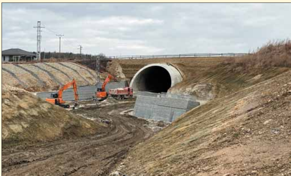
Obr. 6 Gabiony na vjezdovém portále Fig. 6 Gabions at the entrance portal
