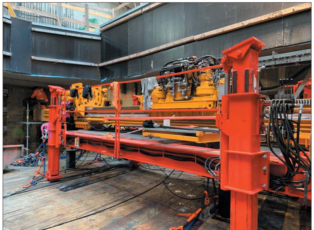
Obr. 8 Zmrazovacie zariadenie tubusu stanice Matzleinsdorferplatz Fig. 8 Freezing equipment for Matzleinsdorferplatz station
