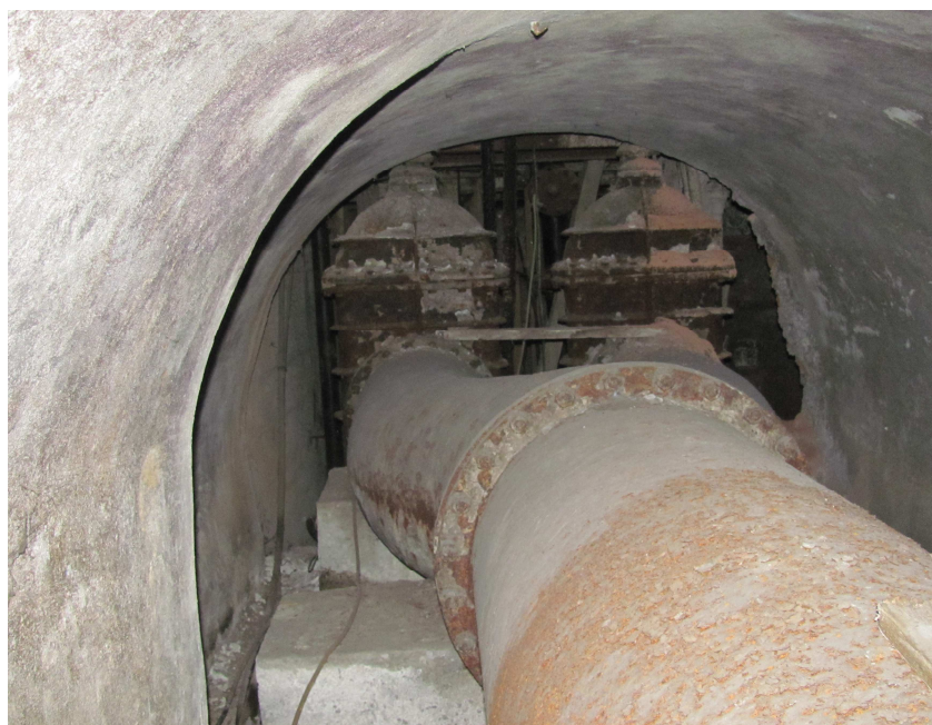
Obr. 3 Nohavica z DN 700 na 2 x DN 500 a 2x šupátka DN 500 mm Fig. 3 Pants made of DN 700 to 2 x DN 500 and 2 valve DN 500 mm
