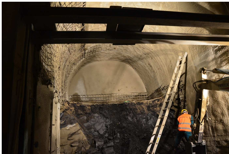
Obr. 7 Chodba CH1- ražba dna Figure 7 Driving of the corridor CH1
